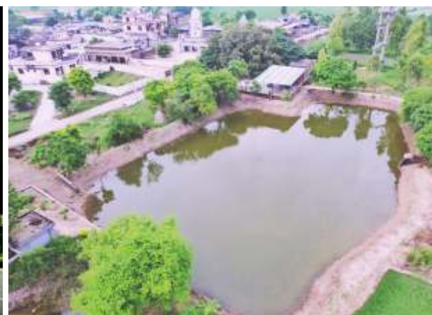
Rehabilitation of pond at Village Jodhpur, Distt. Fatehgarh Sahib
