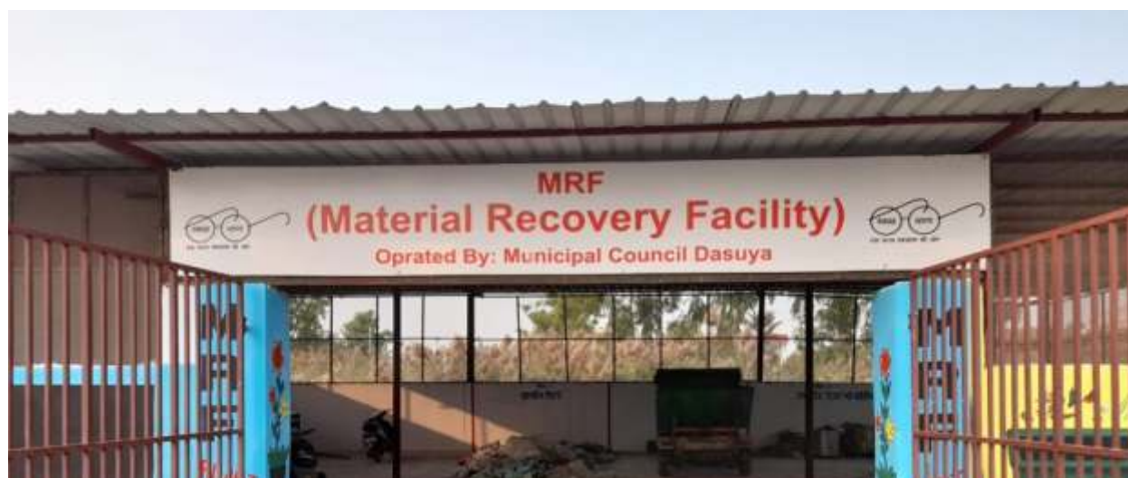
Material Recovery Facility at Dasuya, Distt. Hoshiarpur
