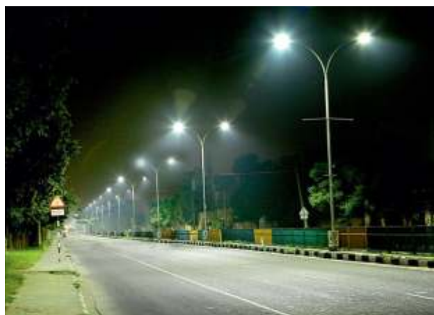
Energy efficient street lighting by PEDDA at Mohali
