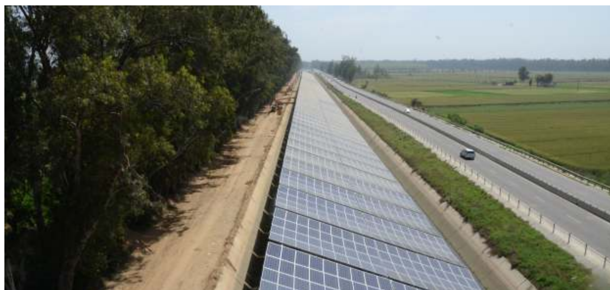
Rooftop Solar Plant at Sidhwan Canal, Ludhiana
