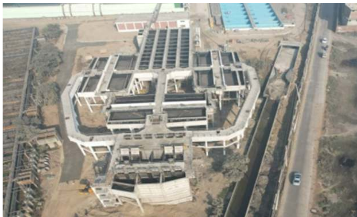
225 MLD STP at Jamalpur, Ludhiana
