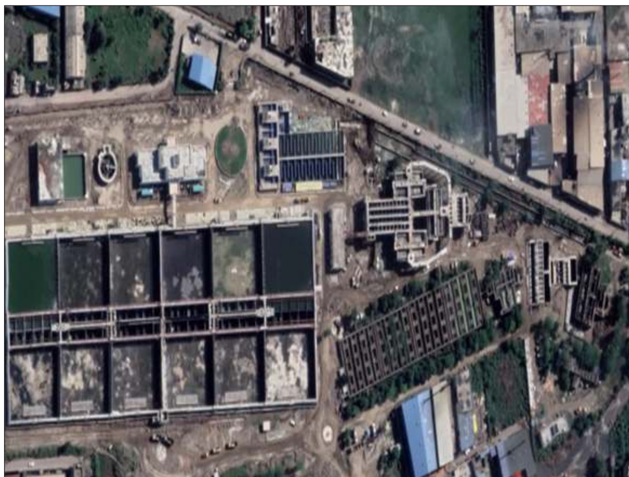
225 MLD STP at Jamalpur, Ludhiana
