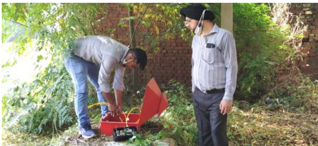
Piezometer installation to monitor ground water level by Department of Water Resources
