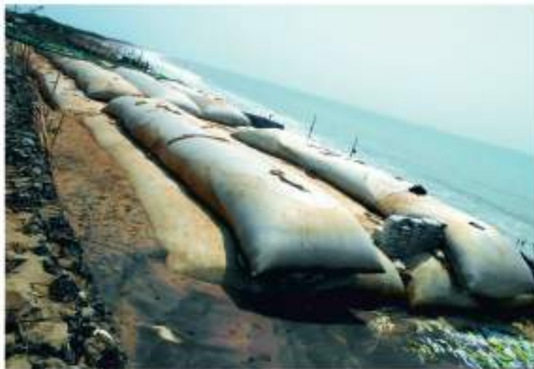
Geo-Synthetic Tube Installation at Pentha, Kendrapada
