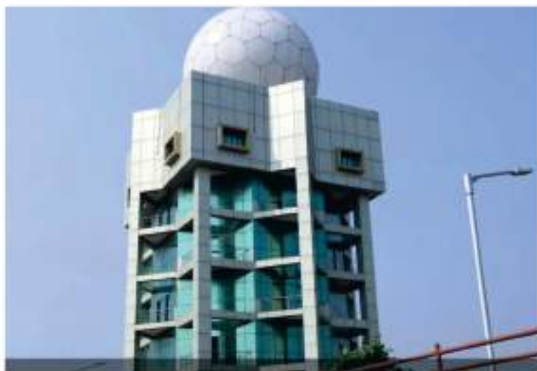
Doppler radar installed at Paradeep
